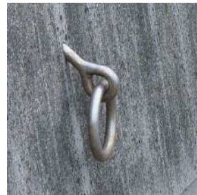
C007B施工写真
